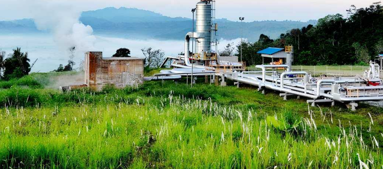
Ulubelu geothermal area, Lampung, Indonesia (source: Pertamina Geothermal Energy)
